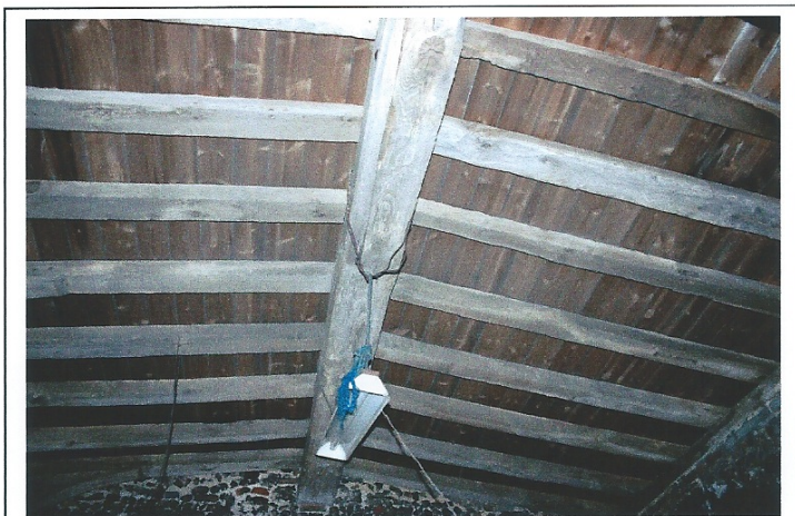
Fig 12: Detail of belfry ceiling
