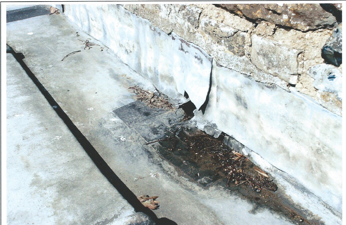
Fig. 19: Tower roof guttering, north side
